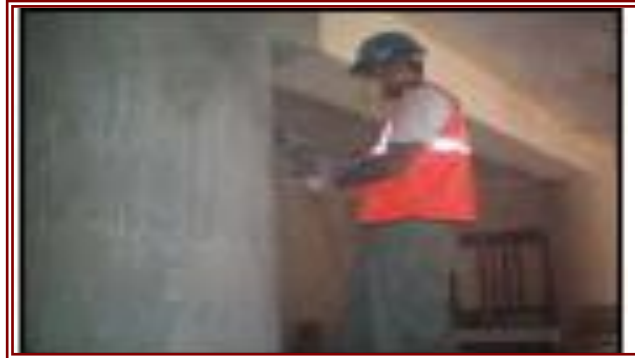
COLUMN UNDER GRINDING
