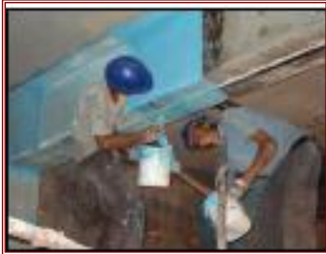
Applying of Epoxy
