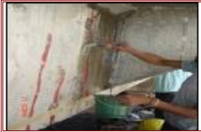
Applying Primer on Beam
