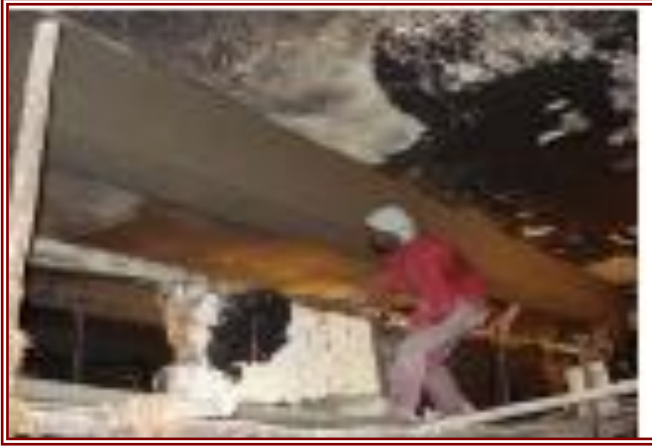
Before Fiber Wrapping
