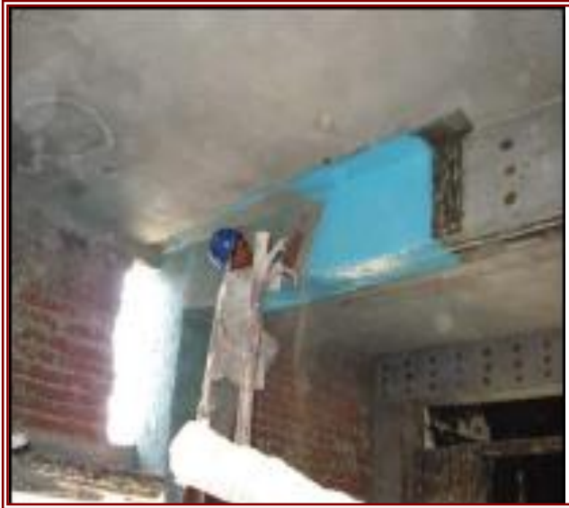
Sprinkling of Sand
