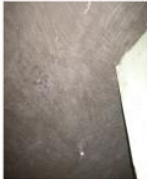
After Applying Polymer Modified Treatment
